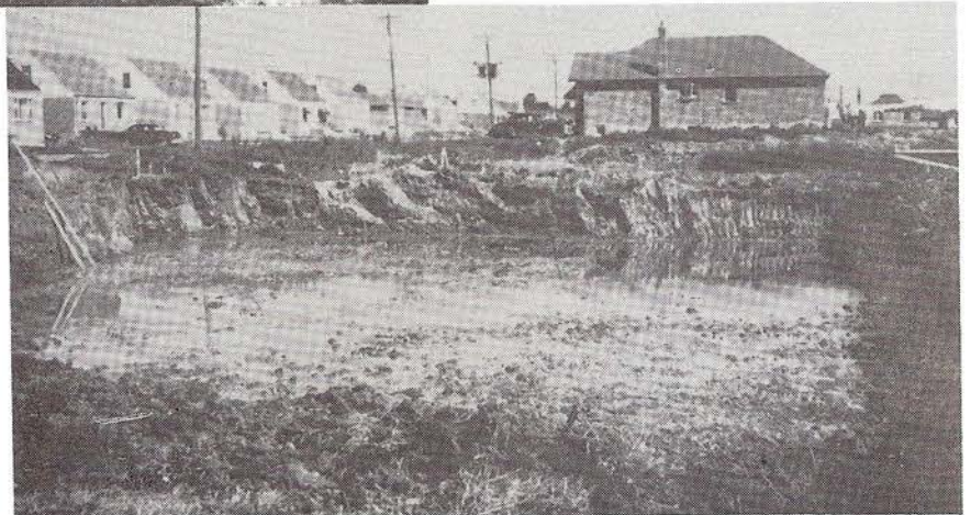
Hole complete, ready to start foundation forms
