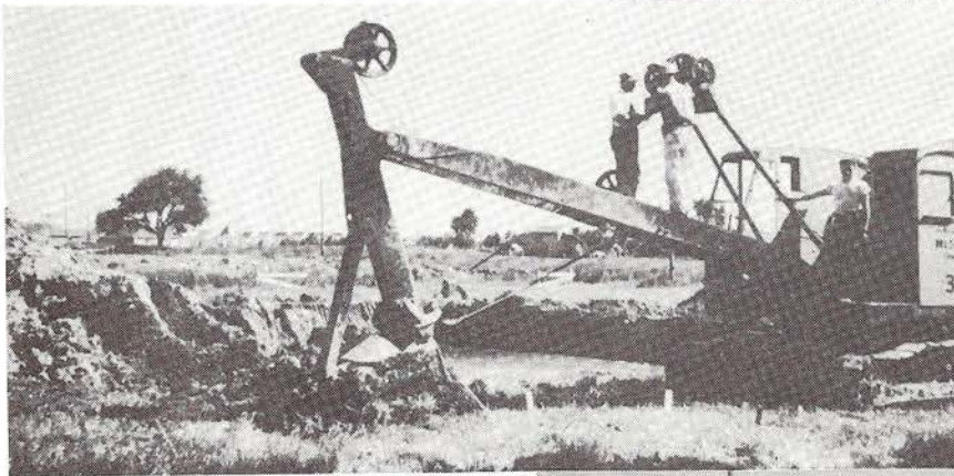
Steam shovel digging hole
